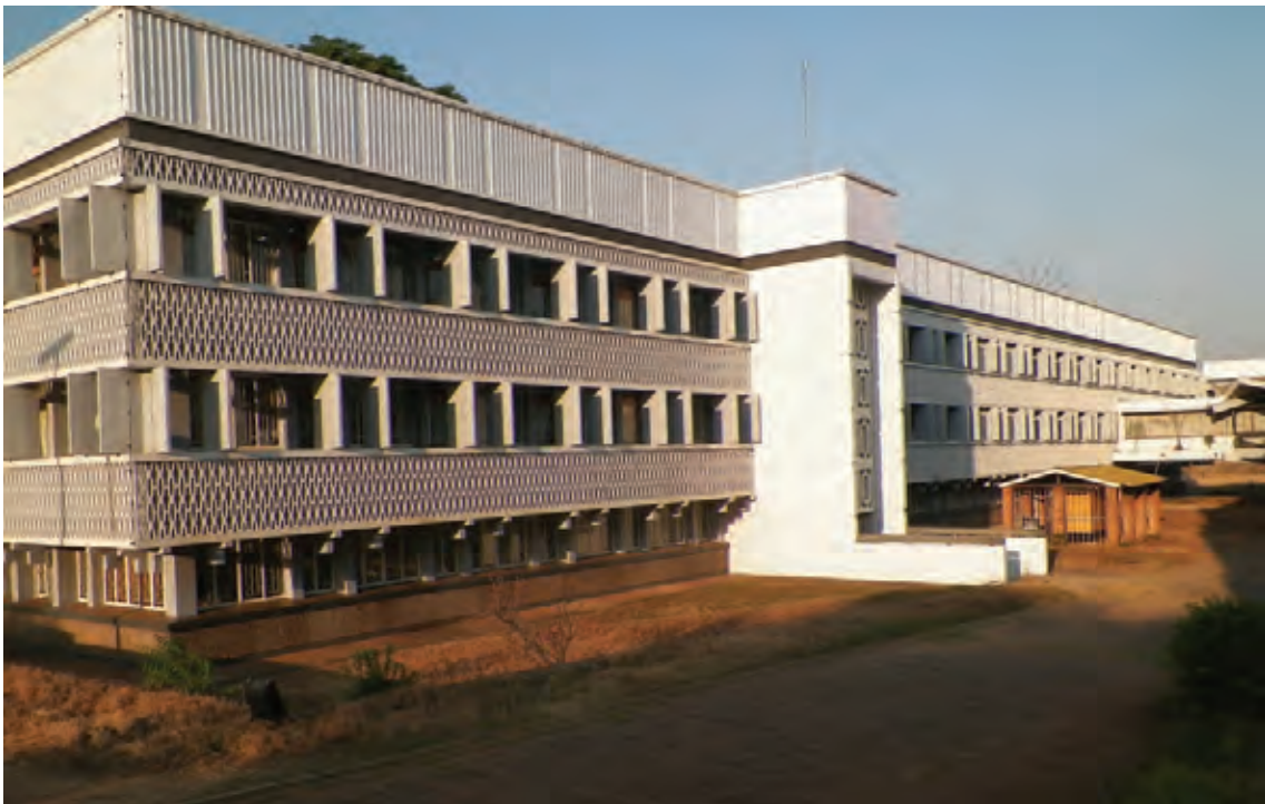
Capital Hill Offices
