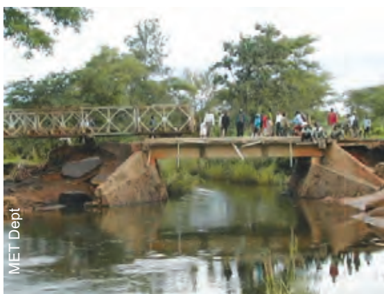
Broken bridge from floods
